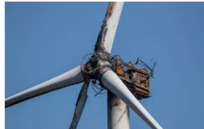
Fire damaged wind turbine to be removed ... saltwire.com
