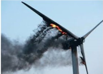
FAILURE OF GEARED WIND TURBINES ... sites.google.com
