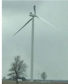
Wind turbine damaged... wind-watch.org
