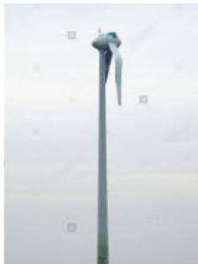
Damage to wind turbin...
