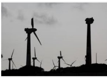
Ignore Puerto Rico Wind Turbine Damage ...
