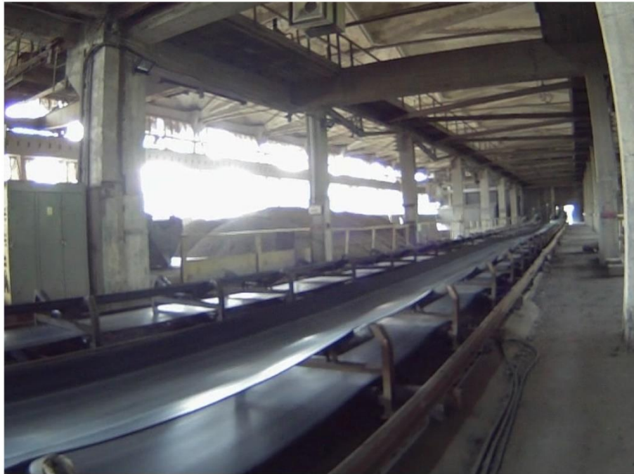
A general view of the belt conveyor in mining sites
